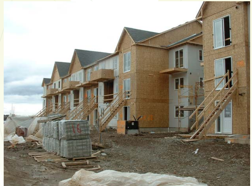
Typical Stacked/Back-to-Back Townhouse Block
