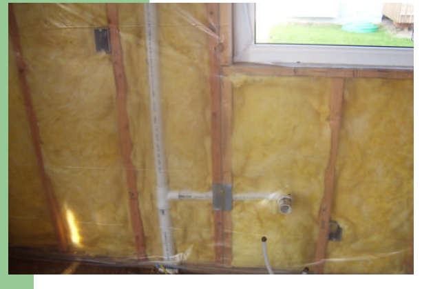
Splitting of Batts
